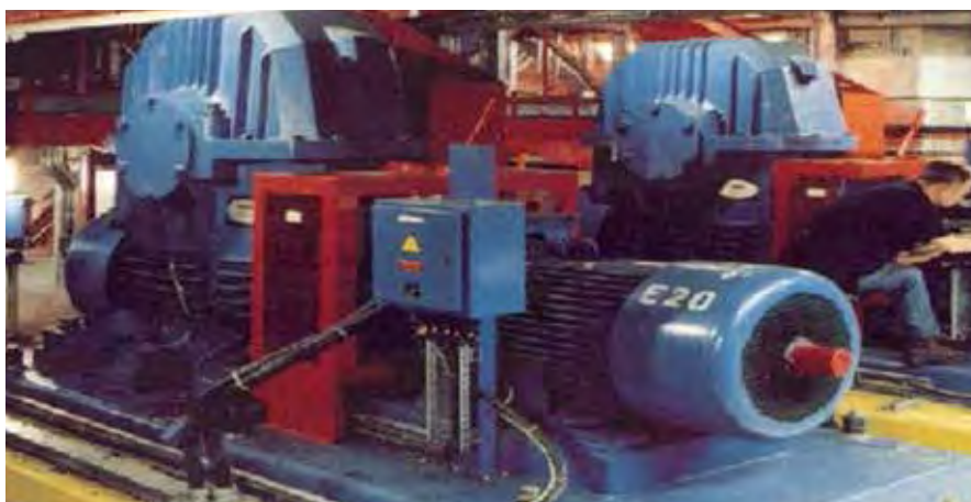
Traditional drive installation at London Underground.
