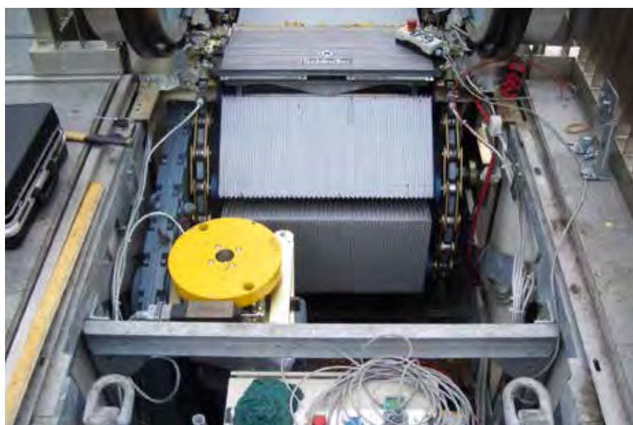
A single-input direct drive installation.
